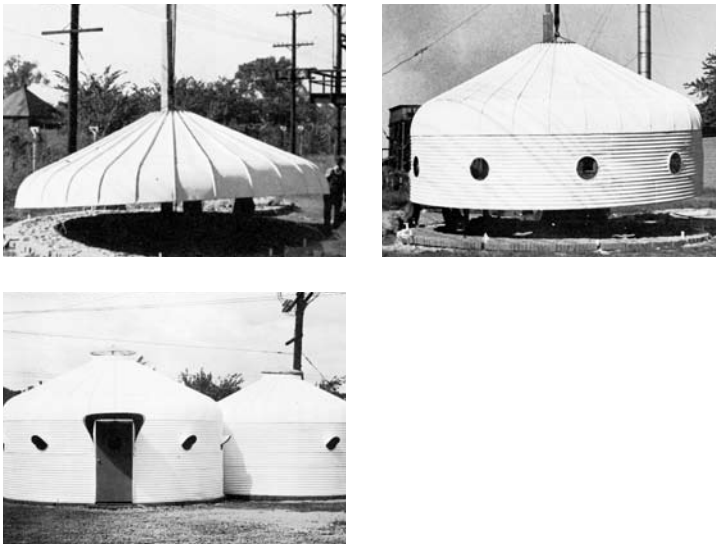
Figs. 2a–c: Richard Buckminster Fuller: Dymaxion Deployment Unit, 1940. Source: Marks 1969, pp. 116–18.
